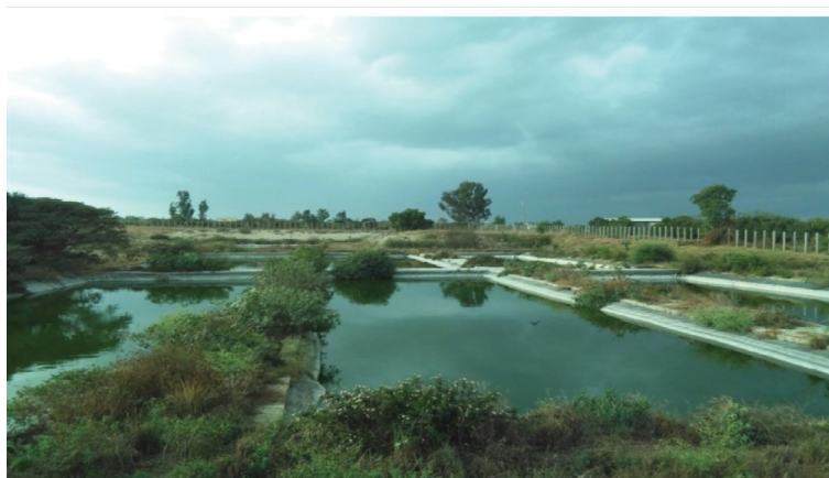
Figure 1. Improperly functioned treatment plant/oxidation ponds. (Source: Image from Ethiopia)
