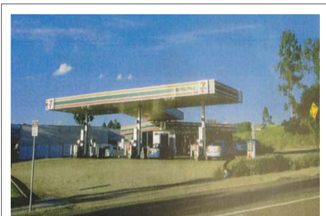
Figure 2. Frontal view of the service station that is to be decommissioned.
