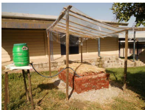
Figure 1: Zero energy cooling chamber (ZECC) construction.
