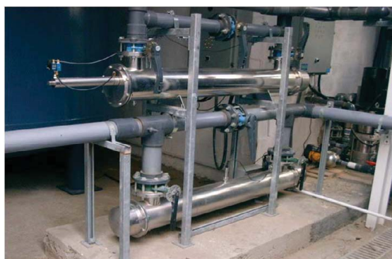
Figure 2: Monitoring Ultraviolet irradiation for deactivating bacteria in Zam Zam water (Careem 2005).
