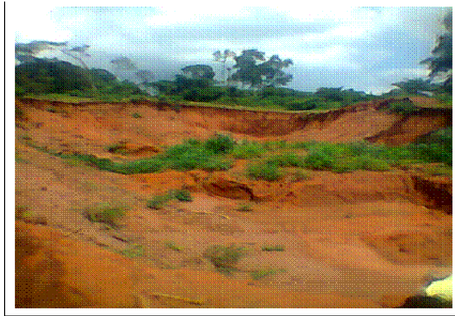
Figure 3. Overview of the Ugwu Orlu Borrow pit
